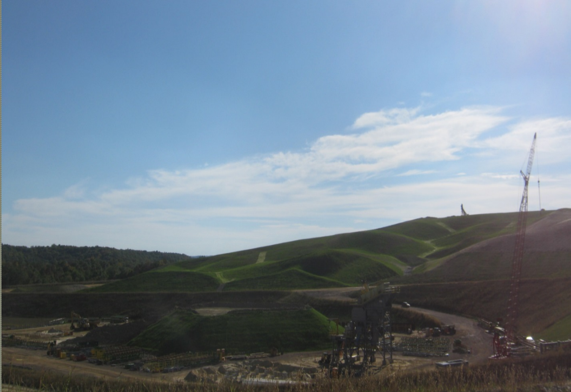
Post Construction View of the “Pickle Park” Geomorphic Land Reclamation Project Looking South-West
