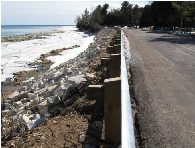
Photograph 1-2. This photograph is looking in an southerly direction and shows the repair of the collapsed left lane of Frogtown Road.
