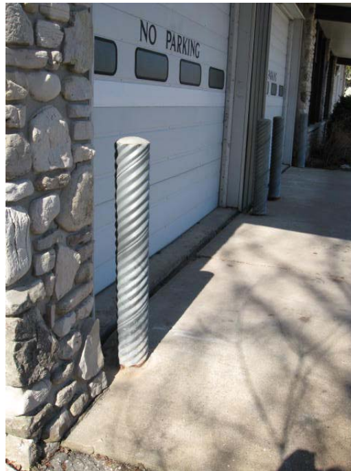
Picture 3-2. The cement driveway approach apron on the north side of the Sister Bay/Liberty Grove Fire Department station at 275 East Mill Road in Sister Bay is migrating to the north away from the building.
