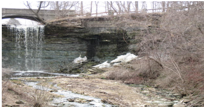
Photograph 13-4. The rock layers under the middle snow pile represents the 2008 rock fall.
